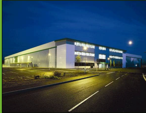
ProLogis Warehousing, Dunstable
